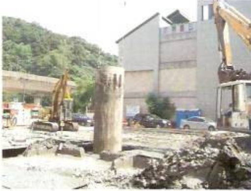
Install casing underground
