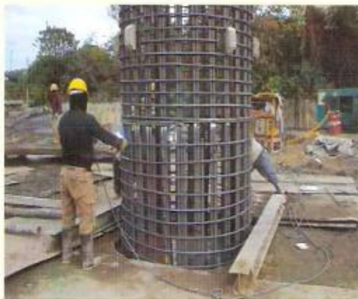
Placing reinforcement cage
